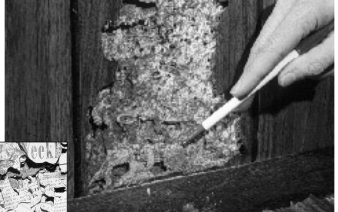
Figure 3-7. Termite-damaged paneling.
