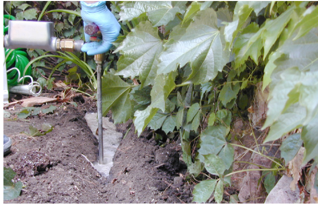
Application outdoors — filling trench
