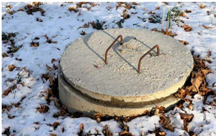
helps to serve as a natural insulator. Some newer septic tanks are installed with a layer of styrofoam-like or other similar insulation on the lid of the tank. Natural or added insulation may not be enough to protect the system when “normal” turns to “extreme.”
