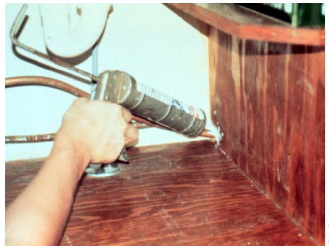
Figure 5-9. Use caulk to seal cracks and crevices and void areas to eliminate these cockroach hiding places.
