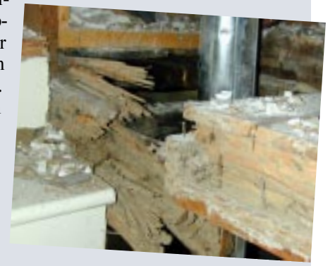
Termite swarms (above) in a Lincoln home with an extensive termite infestation. There was more than $30,000 of damage to the house, including a destroyed house beam (below).
