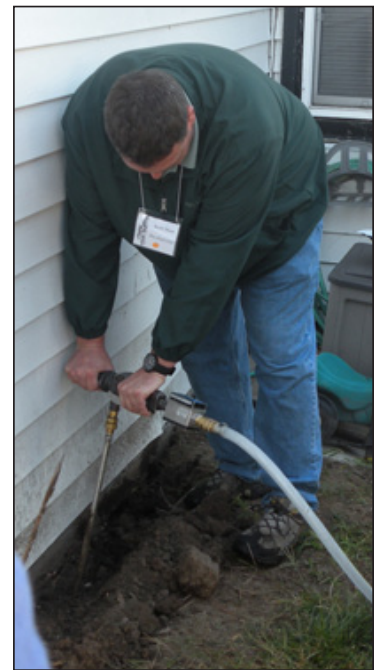
Participants had a chance to practice injecting liquid for a perimeter application.
