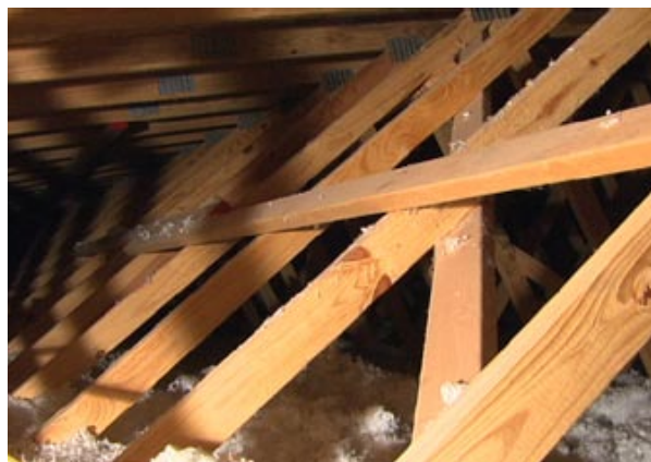
Additional bracing and support reinforces roofs and can prevent wind damage.
