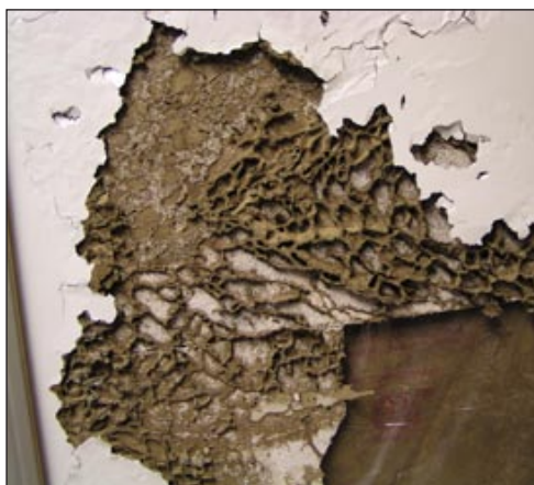
Figure 1. Termite “mud” behind wall paint.
