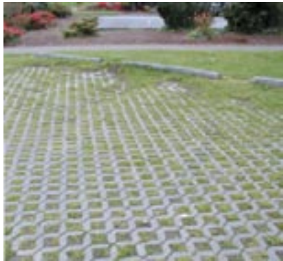
Porous (permeable) pavement allows rain to permeate the soil and gravel layers below.
