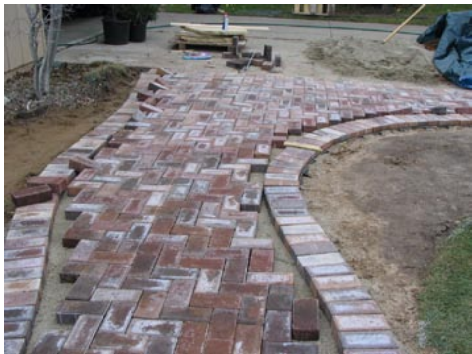
Concrete pavers come in uniform sizes and shapes are relatively easy for a homeowner to install and can replacement for concrete in your landscape.
