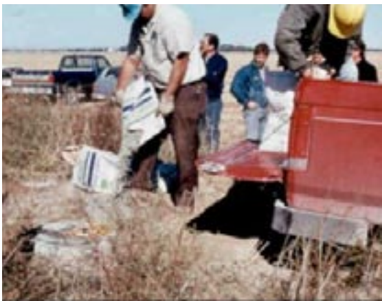
Decommissioning an illegal well includes filling and capping the hole.
