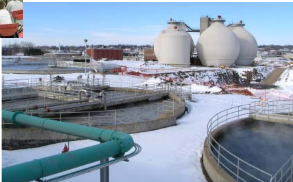
The Theresa Street Wastewater Facility, southwest of 27th and Cornhusker cleans wastewater and produces biosolids 24 hours, 7 days a week and never shuts down for holidays. This facility is currently undergoing major construction to increase capacity to keep pace with Lincoln's increasing population.
