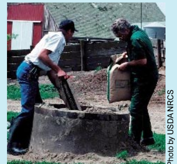
An abandoned well is closed off.
