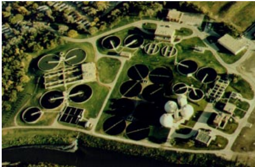
(Fig. 1) Lincoln's biosolids are processed at the Theresa Street Wastewater Facility to make this fertilizer safe for land applications.
