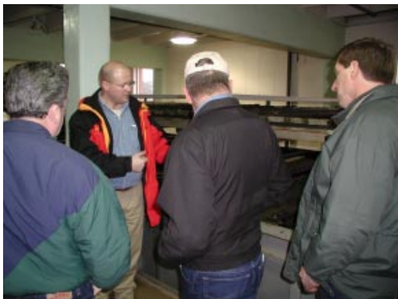
(Fig. 2) Marshall Coleman, Assistant Superintendent of Wastewater Operations, describes to workshop attendees the process used to thicken waste-activated sludge prior to being pumped to the egg-shaped anaerobic digesters.
