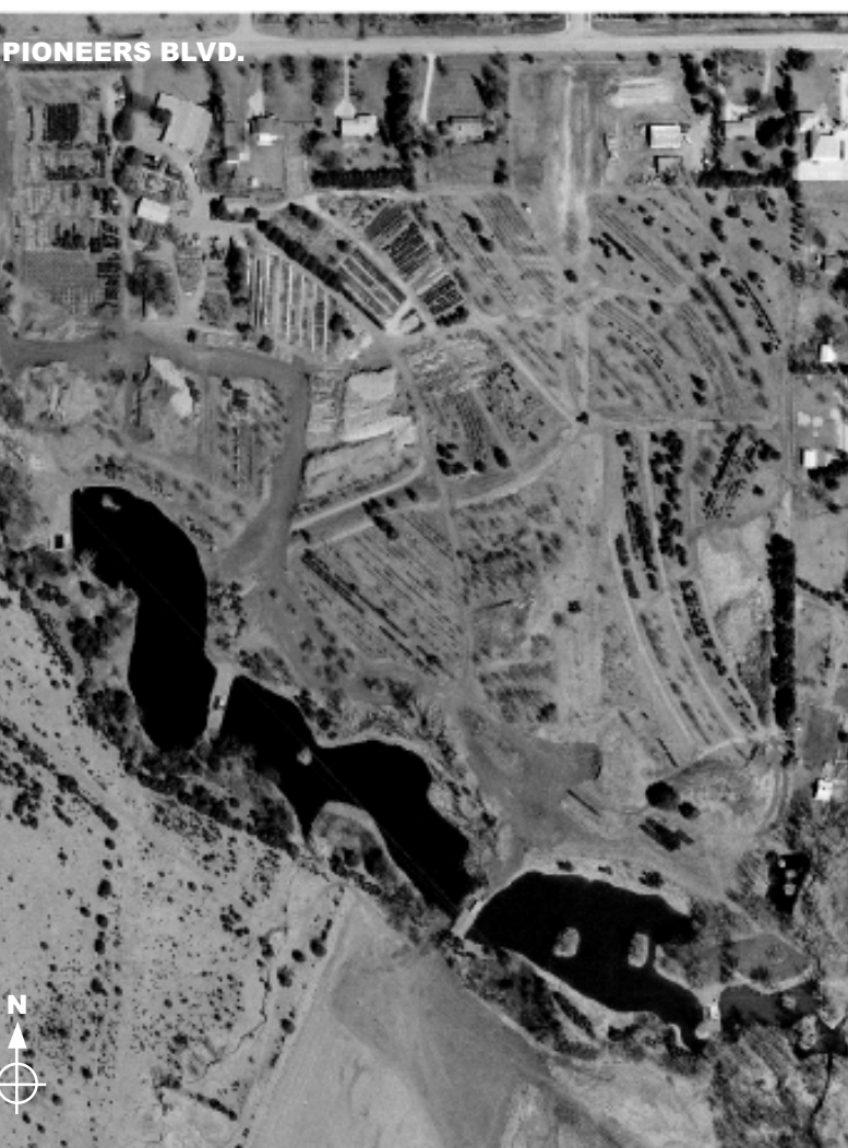
The Antelope Commons Constructed Wetlands (above) was the centerpiece of the Holmes Lake Sub-
