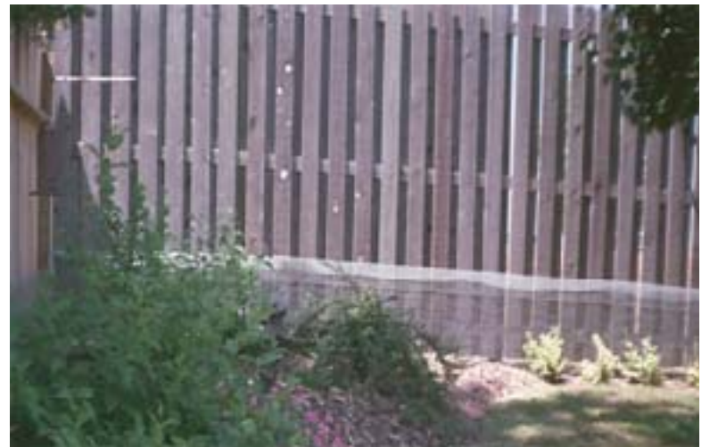
A rabbit fence added to an existing fence.
